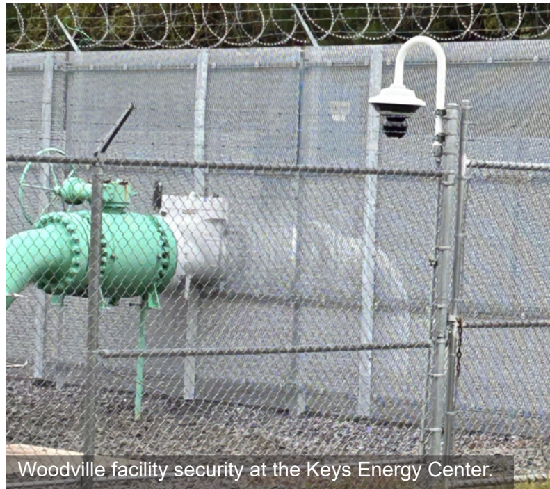
The Keys Energy Center Woodville facility pig launcher from which in-line smart tools are launched.
