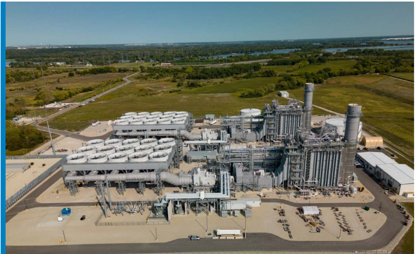
Photo: CPV Three Rivers, a facility subject to NSPS KKKK, is located in Morris, Illinois. The facility's ownership is split equally among Osaka Gas USA, Concord Infrastructure Investments, Harrison Street, and Axiom Infrastructure. CAMS provides O&M services.
