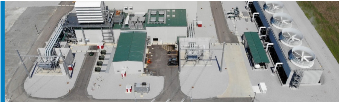
Photo: Middletown Energy Center
