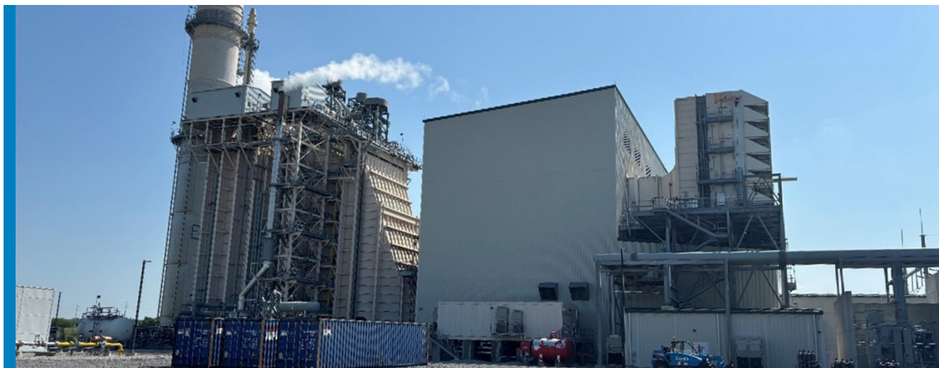
Photo: Middletown Energy Center – Enclosed turbine configuration
