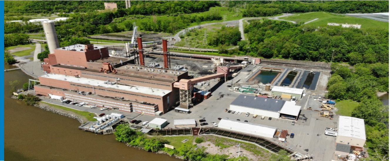
Photo: Danskammer Generating Station, Newburgh, NY. Danskammer is a 491-MW combined-cycle natural gas-fired power plant owned by Tiger Infrastructure and operated and managed by CAMS.
