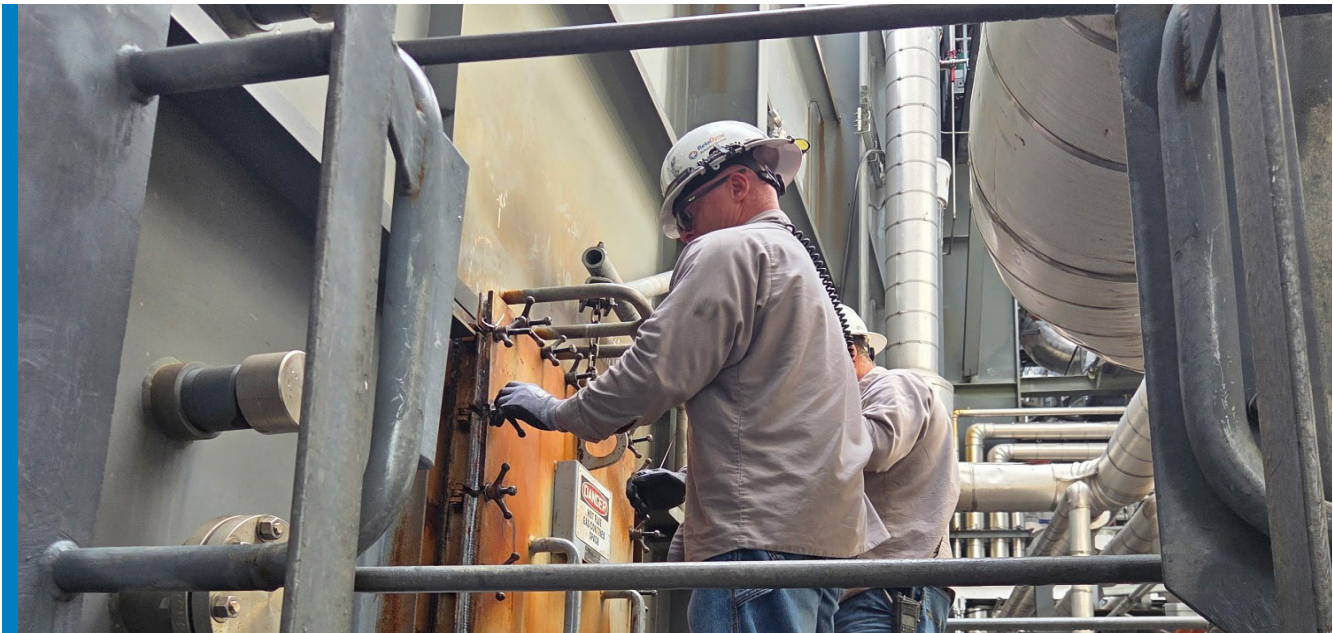
Photo: CAMS employees close a confined space after work was completed.
