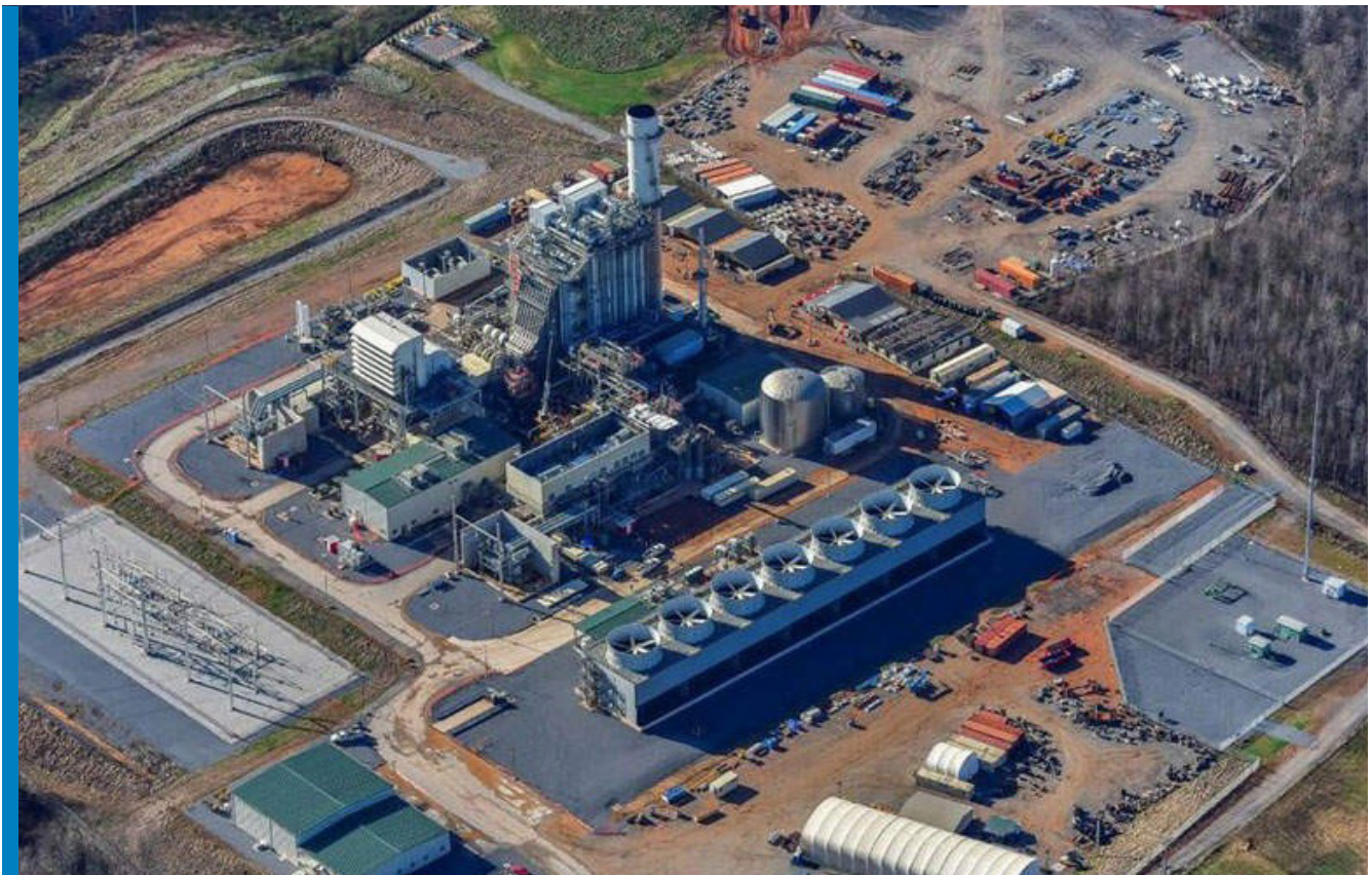
Photo: The Kings Mountain Energy Center combustion turbines are subject to 40 CFR Part 60 Subpart KKKK. Kings Mountain is owned by Carolina Power Partners, LLC and is operated and managed by CAMS.
